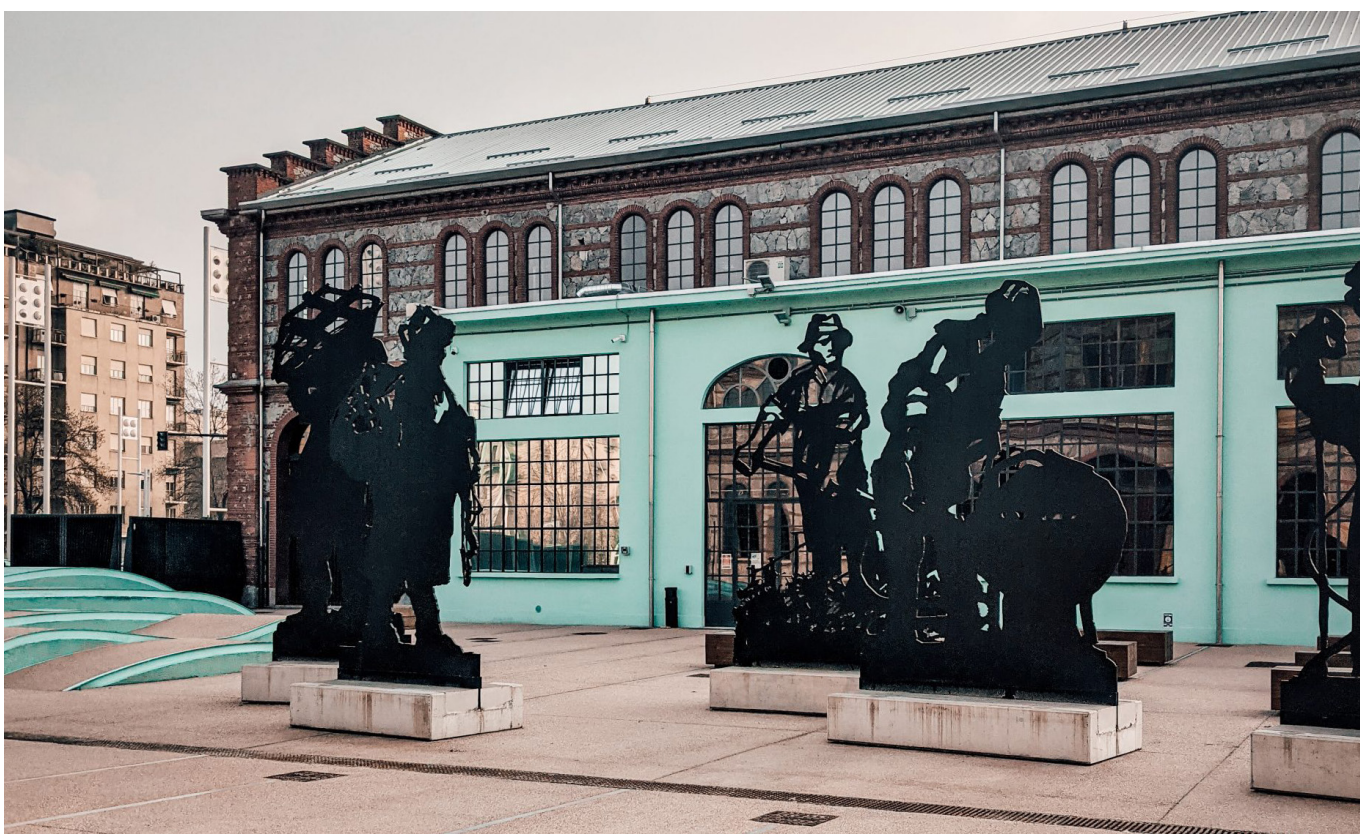
Restructuration et redressement d'O.G.R. de Turin, pentes de toit en panneau Lithos 5 Isolpack. Restructuring and recovery of O.G.R. of Turin, roof pitches made with Lithos 5 Isolpack panel.
