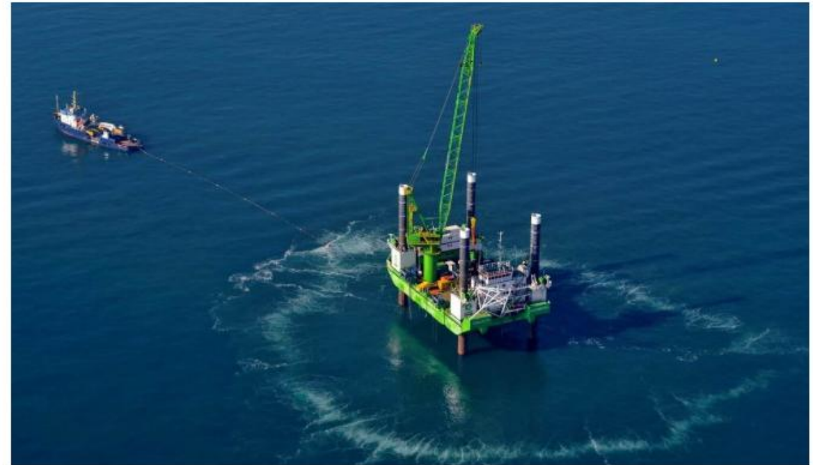
Pile driving operation with bubble curtain. © Trianel/Lang
