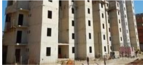
U \sim 3.5 \text{ W/m}^2.\text{K} Monolithic concrete wall
