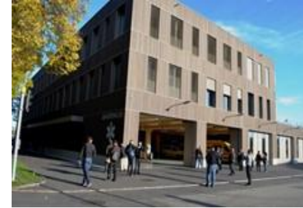
“sustainable” architecture 15-40% window to wall ratio, bioclimatic design approach, natural/hybrid ventilation, external movable solar protection, radiant cooling
