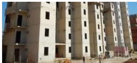
U \sim 3.5 \text{ W/m}^2\cdot\text{K} Monolithic concrete wall
