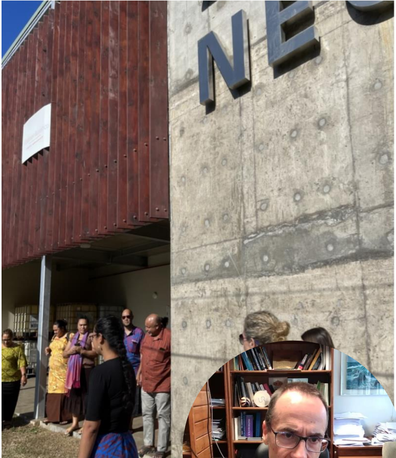
Early Warning Centre
